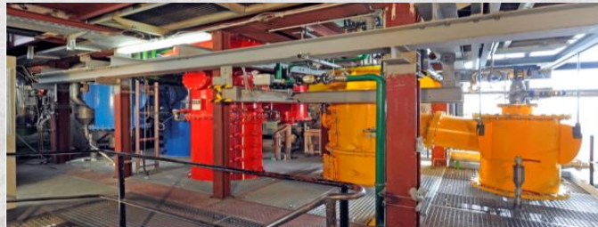
Alstom Power Calcium Looping – TRL 3
